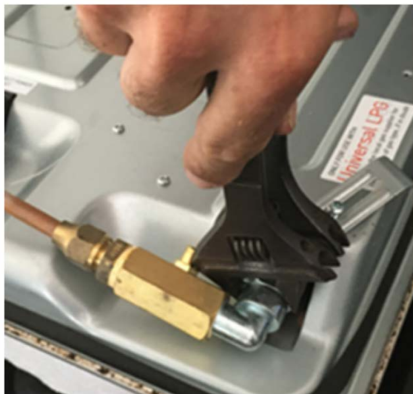
Image 1a - Domestic kitchen elbow assembly
