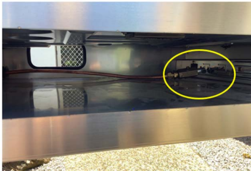
Image 2a - Failed connecting elbow in recreational vehicle
